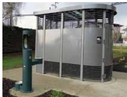
Portland Loo at the West Bay Walkway.
