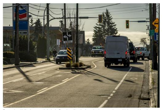
Example of bike lane on Admirals Road ending before the intersection, which provides the person cycling with no protection from the vehicle. According to the BC Active Transportation Design Guide, a green conflict zone marking should be provided for the bicycle lane up to the intersection.
