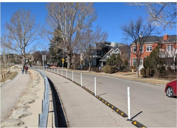
Example of a protected bike facility in Kelowna, BC with quick-build materials including flexible delineator posts and a rubber curb.
