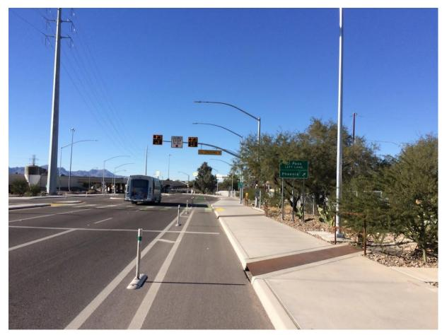
Example of a quick-build cycling facility in Tucson, Arizona that has delineator posts as the separation material. This is the type of facility envisioned on Tillicum Road / Lampson Street as part of the quick-build network.
