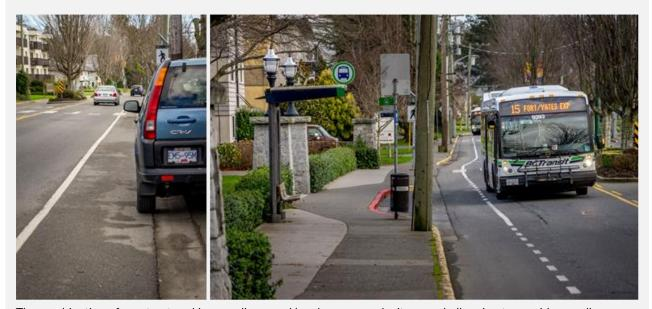
The combination of on-street parking, medians, and bus layovers make it more challenging to provide a cycling facility with full protection for all sections of the Esquimalt Road corridor.
