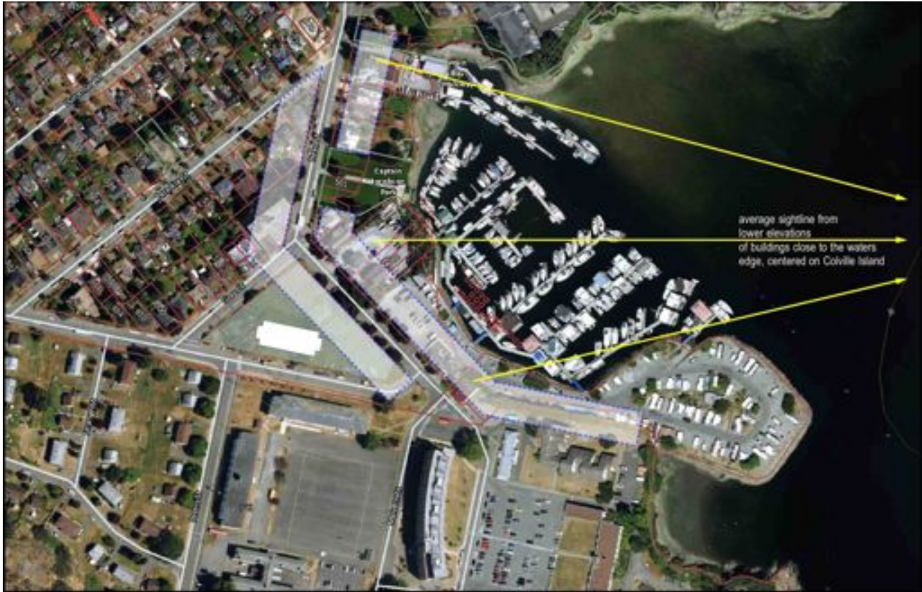
At the ocean's edge, in the area of 2 storey buildings, the sightlines are towards the interior of the cove, and centered on Coville Island.
