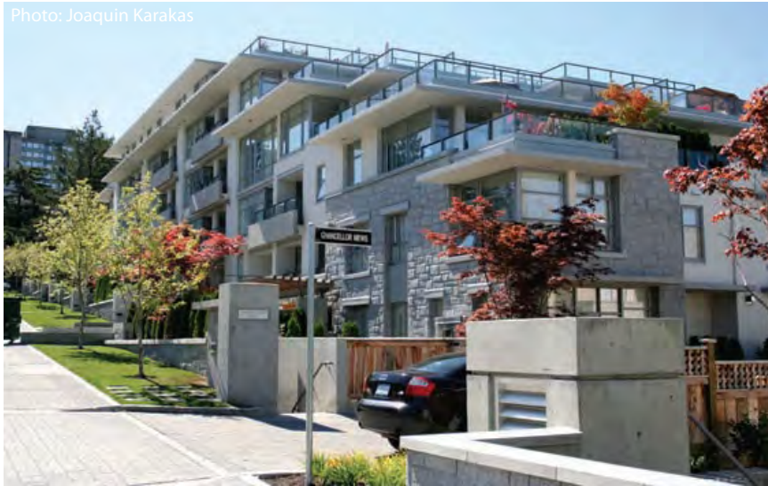
This building steps down to the slope to reduce the visual impact from it's massing
