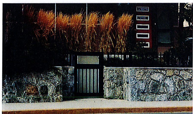
Retaining wall and low metal fence at 1060 Tillicum Road
