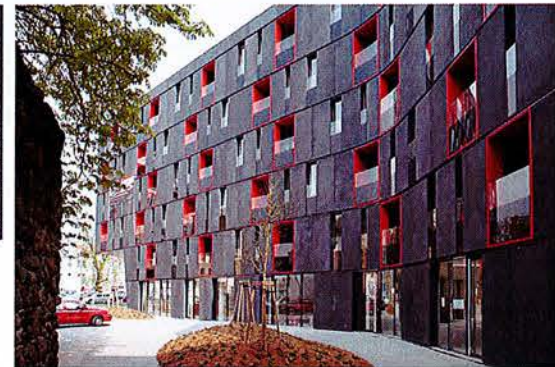
Ostrava City Gate by Kuba & Pilaf Architekti
