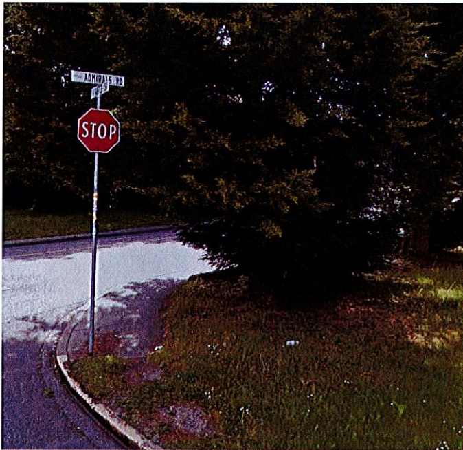
Figure 4.1: Vegetation Obstructing Visibility at the Admirals Road / Astle Street intersection
