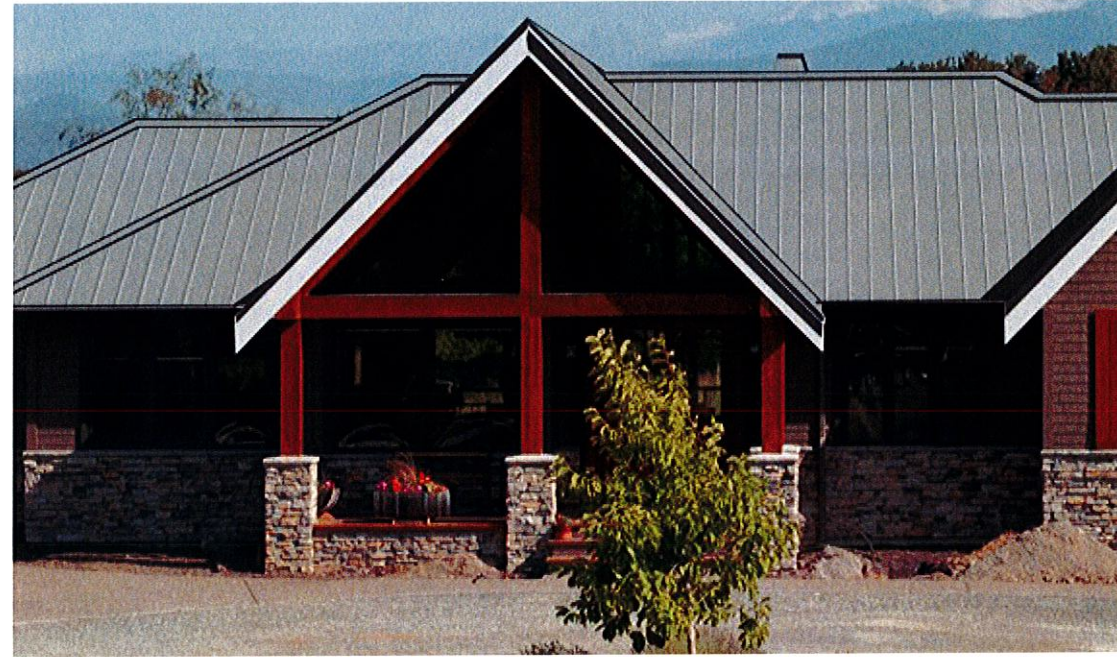
ROOFING TO BE WESTFORM METALS PROLOCK SHEET METAL ROOFING IN REGENT GREY IN 24 GAUGE, AS PICTURED ABOVE.
