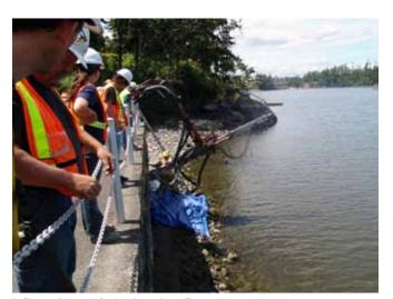
Drilling anchors into the Arm Street Seawall
