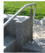
Stainless Steel Handrails
