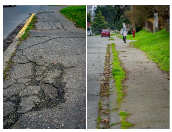
Examples of poor sidewalk condition on Lyall Street with cracking concrete sidewalk (left) and debris / uplift (right).
