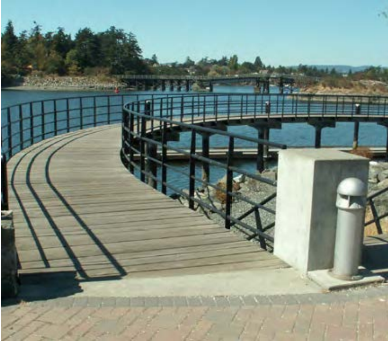
Photo: Franc D’Ambrosio Architecture and Urbanism
