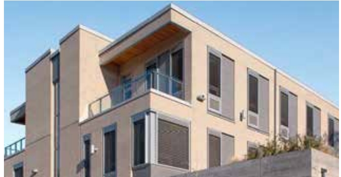
26.6.2 Sun shading should be considered to control heat gain in the summer.
