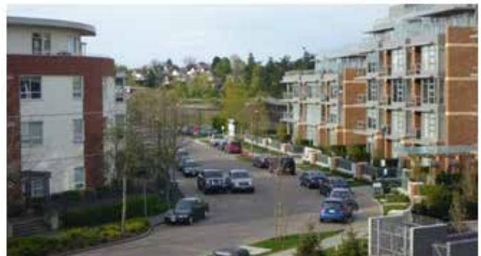
26.6.12 Orient upper-storey windows and balconies to overlook adjoining streets and public space.
