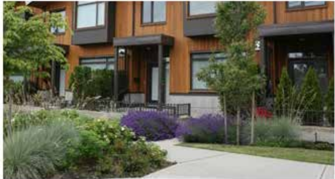
26.6.19 Provide for slightly raised entrances to ground floor residences along with private yards that are accessible from the fronting street or lane to encourage community interaction.
