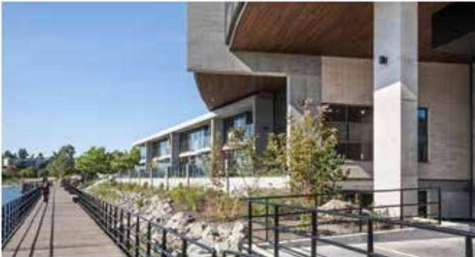
26.6.18 Provide for building occupants to overlook public streets, parks, walkways and spaces, considering security and privacy of residents.
