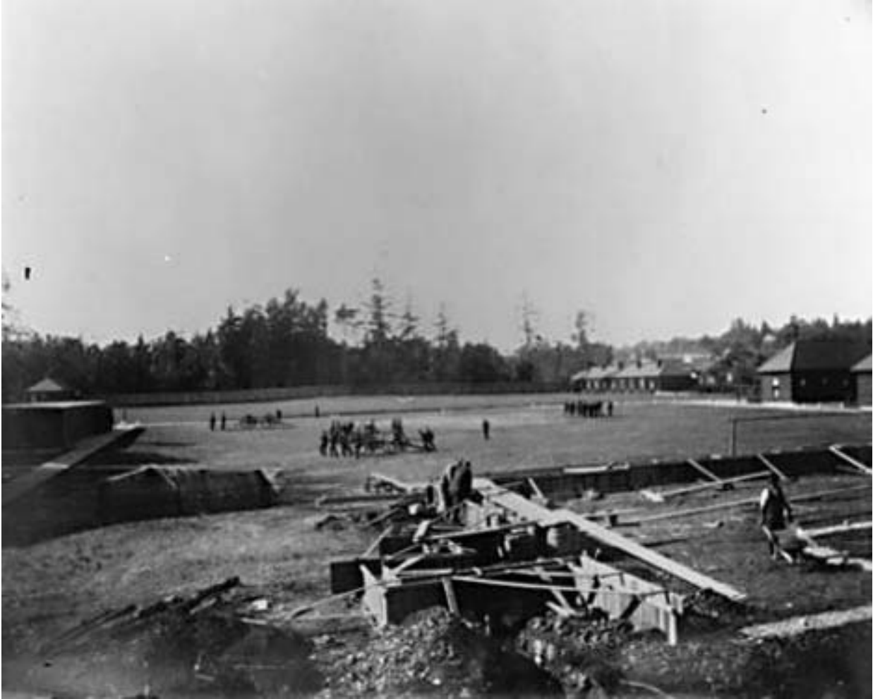
Work Point, looking west over the construction of the "Works Office" at Work Point Barracks circa 1893. In the background are the Royal Marine Artillery with their muzzle-loader carriage guns in the Parade Square and the Enlisted Men's Barracks to the far right. [Young Collection, Esquimalt Archives 994.4.7]
