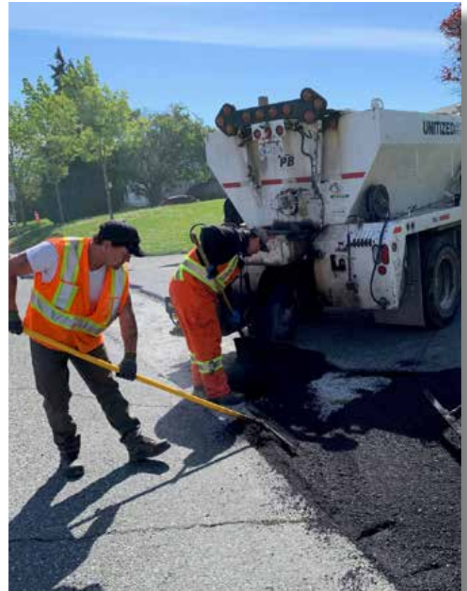
Crews repair and repave roadways in Esquimalt.
