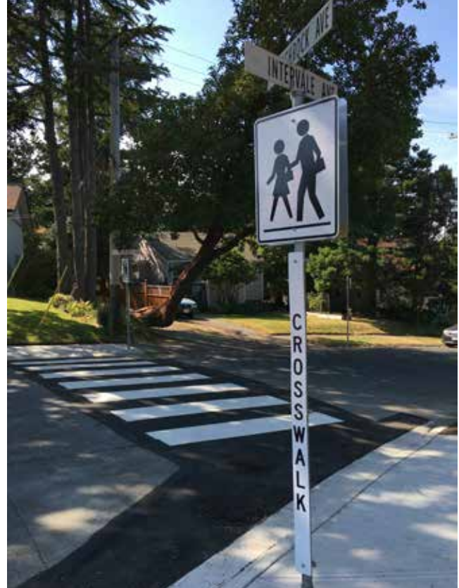
Crossing improvements at Intervale Ave and Highrock Ave, including fresh paint, new curb ramps and signage.
