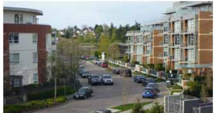
12. Orient upper-storey windows and balconies to overlook adjoining streets and public space.
