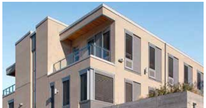
2. Sun shading should be considered to control heat gain in the summer.
