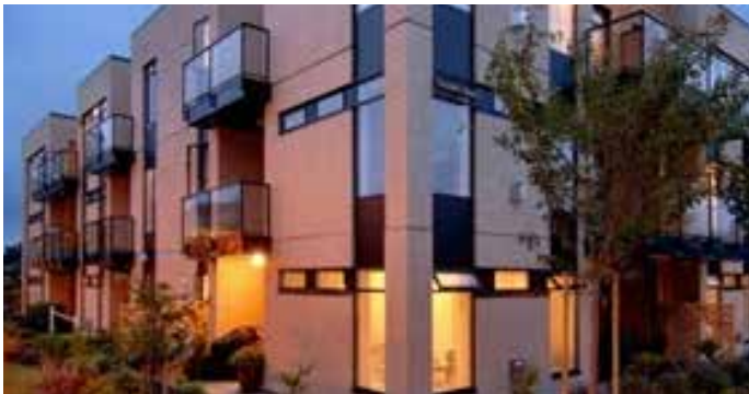
22. All exterior lighting should avoid excessive stray light pollution and should meet International Dark-Sky standards.
