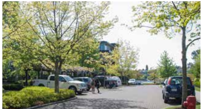
23. Wherever possible, outdoor storage and parking areas should be screened from view.
