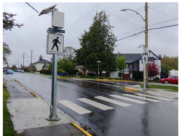
New Rectangular Rapid Flashing Beacon (RRFB) crosswalk on Lyall St. at Paradise St.
