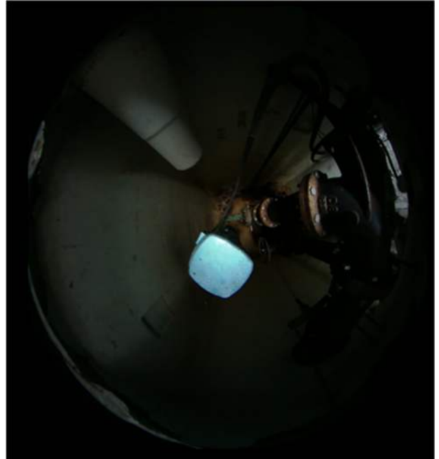
Figure 6 - Uganda PS - Pump 1 Bottom Level (1)
