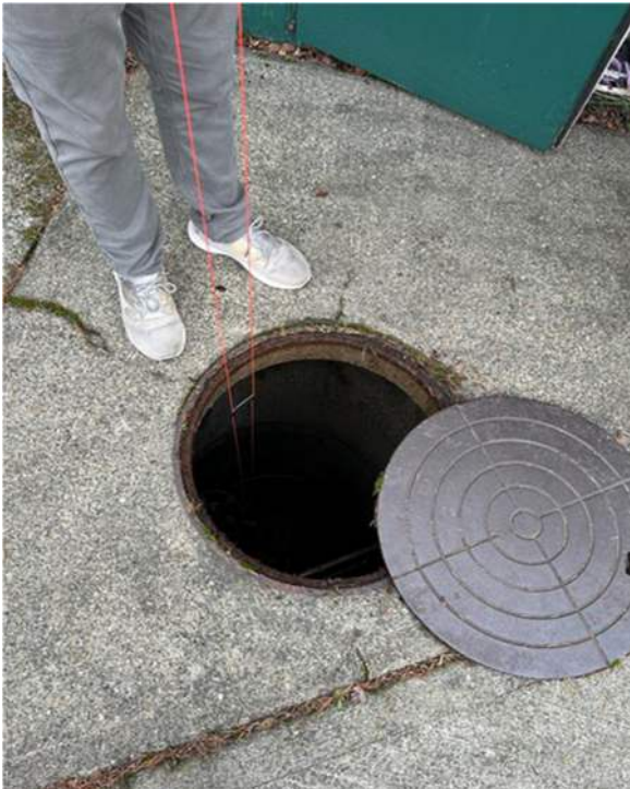
Figure 11 – Uganda PS – Bypass Chamber – Entrance
