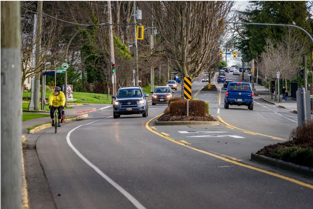
Existing bicycle lane on Esquimalt Road at Fernhill Road. Bike lanes that are physically protected from motor vehicle traffic was among the top desired improvements identified by the community. Section 6.0 identifies improvements to cycling corridors such as Esquimalt Road to make them more suitable for all ages and abilities.
