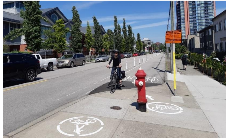
Example of a quick-build cycling facility in Agnes street (New Westminster, BC). This is one of the many projects that have been implemented in the last couple years offering flexibility and adaptability to municipalities and ultimately a cost-effective way to test the appropriate streetscape configuration.
