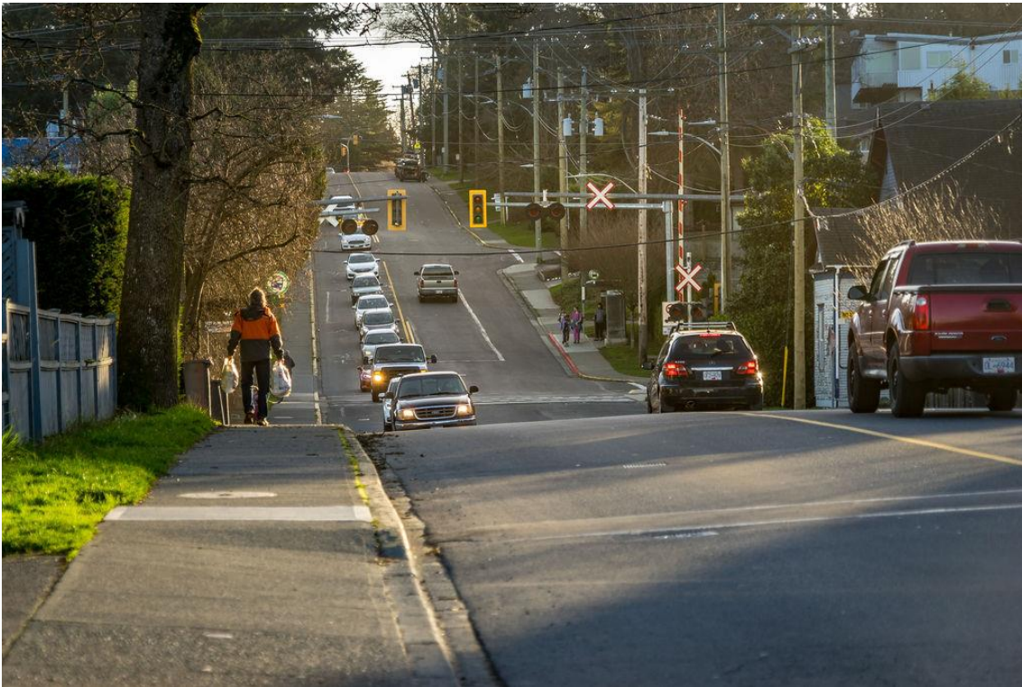
Example of pedestrian walking along Lampson Street with no buffer between sidewalk and motor vehicle traffic. Lampson Street is a Major Road signed at 50 km/h and this section of the road sees approximately, 11,350 vehicles per day, making it uncomfortable to walk on for most pedestrians.
